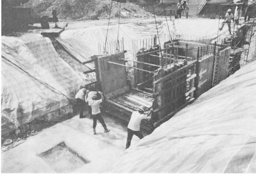
Fig. 2 Precast segments being placed on a prepared bed on the open cut at certain spacing.
