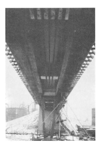
Fig. 2 External application of the prestressing tendons
