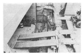
Fig. 2 - Construction of launching bed Fig. 3 - Hydraulic jacks
