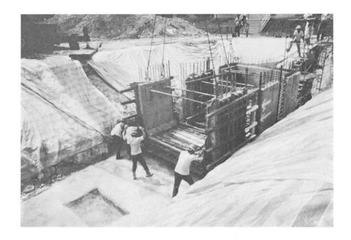
$\underline{\text{Fig. 2}}$  Precast segments being placed on a prepared bed on the open cut at certain spacing.
