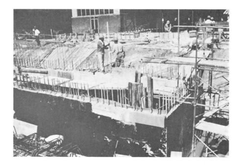
$\begin{array}{c} \underline{\text{Fig. 3}} \ \ \text{End of Phase I.} \\ \text{Water bars have been fixed at joints facing Phase II} \\ \text{cast-in-place concrete.} \end{array}$
