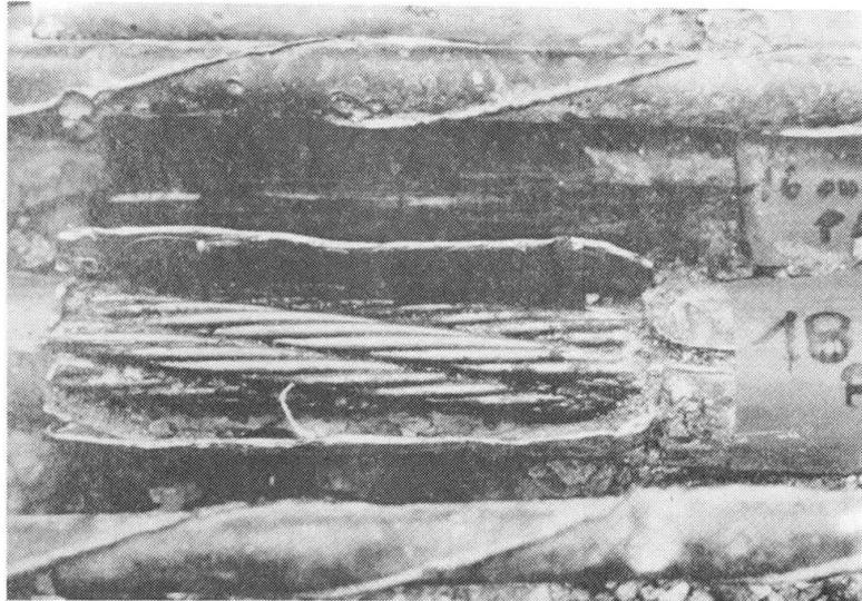
**Fig. 6** : Attack of the tendons by corrosion
