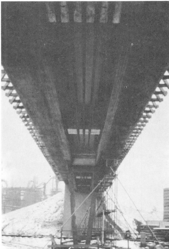
Fig. 2 External application of the prestressing tendons
