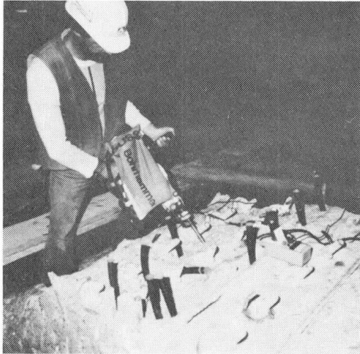
Fig.3 Drill hammer with automatic switch-off
