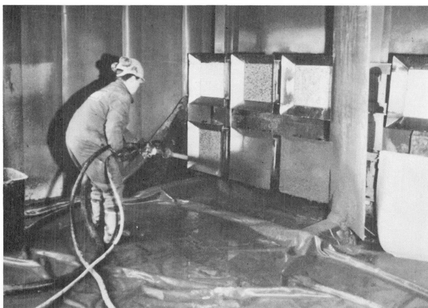
Fig. 1 Shotcrete gunned towards formwork, with bottoms of sawn concrete surfaces.
