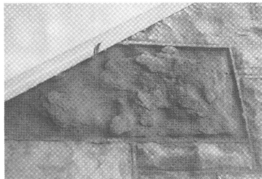
Fig. 1 Stone deterioration at repointed joint
