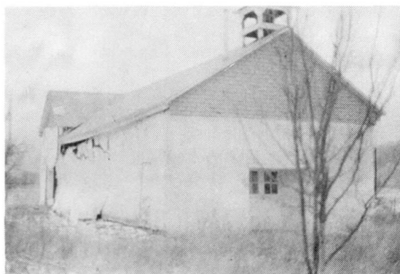
Fig. 4 Wall failure resulting from high moisture content
