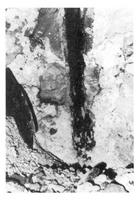
fig. 3 Negative example of protection against corrosion. Reinforcement bar without enough protective cement mortar covering. The diameter of the drill hole was to small.
