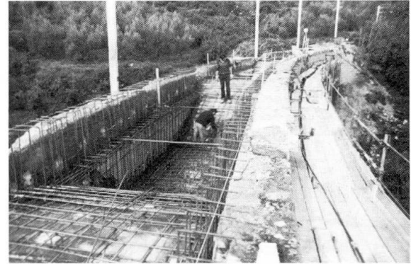
Fig. 26 The realization of a reinforced concrete caisson.
