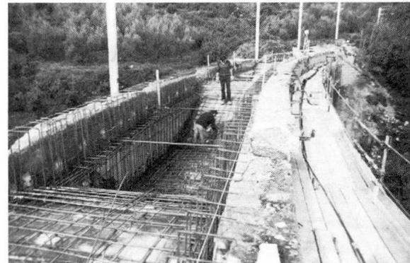
Fig. 26 The realization of a reinforced concrete caisson.
