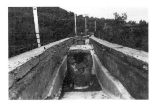
Fig. 25 The lesion in the masonary structures of the bridge.
