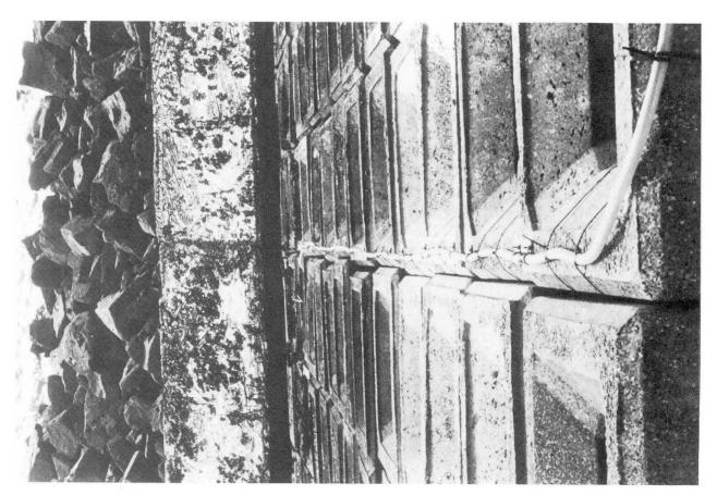
$\underline{\text{Fig. 10}}$  Data cable attached to face of Cob armour units.
