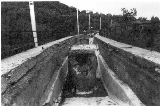
Fig. 25 The lesion in the masonry structures of the bridge.
