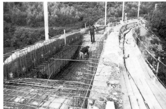
Fig. 26 The realization of a reinforced concrete caisson.
