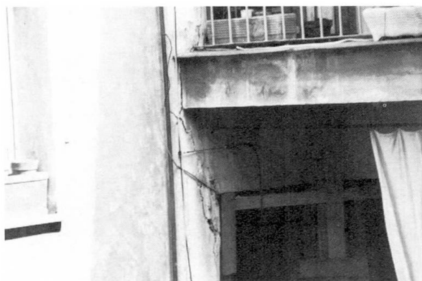
Fig. 8-11 Some of the most significant cracks on the masonry structures
