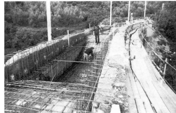
Fig. 26 The realization of a reinforced concrete caisson.
