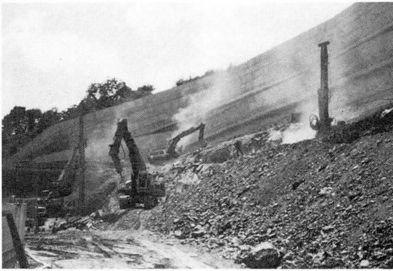
Fig. 18 Service Center in Genova, the retaining structures.
