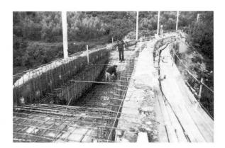
Fig. 26 The realization of a reinforced concrete caisson.
