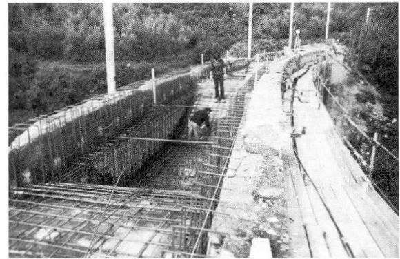
Fig. 26 The realization of a reinforced concrete caisson.
