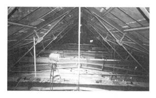
Fig. 12 The steel beams placed at the extrados of the vault of the Major Council Hall.
