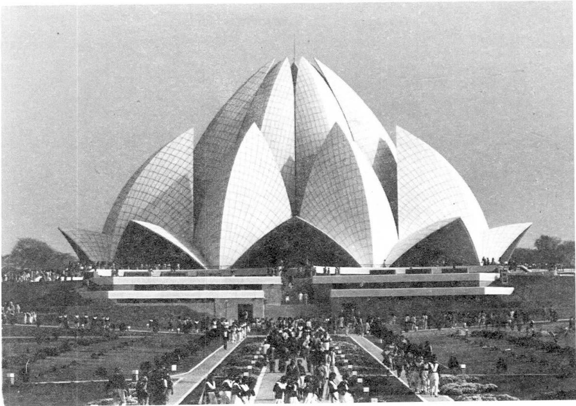
processes were used to manufacture sample panels of exposed concrete. White concrete composed of white cement, silica sand, and dolomite aggregate, was selected.
