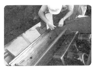
Fig. 5 Checking of mould dimensions
