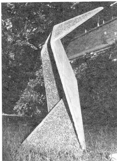
were cast horizontally with open joint lines between them. The mid-plane reinforcing mesh crossed the open joints. About seven days after casting the folding was carried out. The yielded reinforcement forms the hinge along each joint which permits the folding to take place. The joint lines were then filled with mortar to hold the joint rigid.
