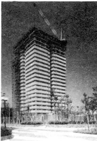
Fig.1 Building under construction
