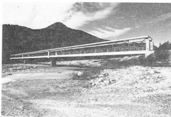
Fig. 10 The Mugnago Bridge spanning (3 x 40,0 meters)
