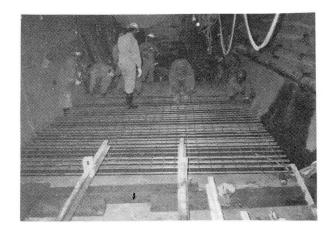
Fig.14 Reinforcements for invert of tunnel
