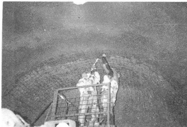
Fig.12 Reinforcing grids for shotcrete
