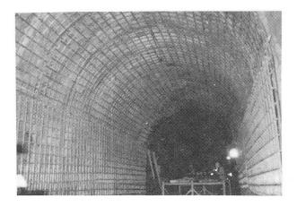
$\frac{\text{Fig.}13}{\text{tunnel}}$  Reinforcements for arch of
