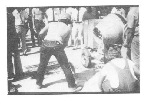
Fig. 3 Placing PC into Repair Area on Bridge
