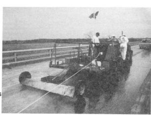
Fig. 4. Polyester Resin Applied by Spray Bar for Construction of Overlay
