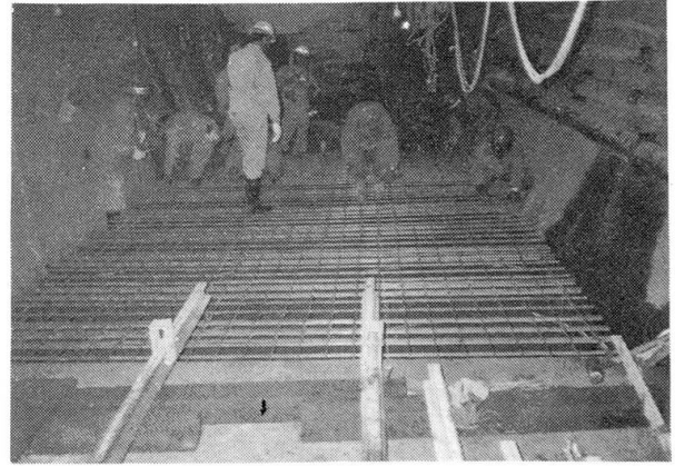
Fig.14 Reinforcements for invert of tunnel
