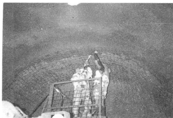
Fig.12 Reinforcing grids for shotcrete
