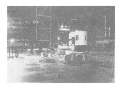
Fig. 6 Floor surface finishing robot
