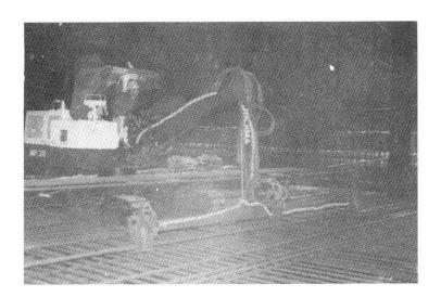
Fig. 8 Rebar arranging robot
