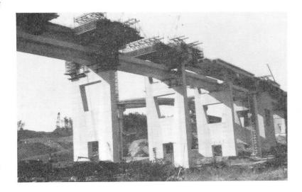
Fig. 2 Construction of Yoshima Viaduct
