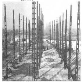
Fig.4. Lifting of two segments of a hospital building with column spacing 6.00x6.00 m, before lifting
