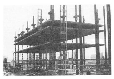
Fig.5. During lifting of first segment
