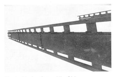
Fig.2. Steel column with slide bars and bearing collars
