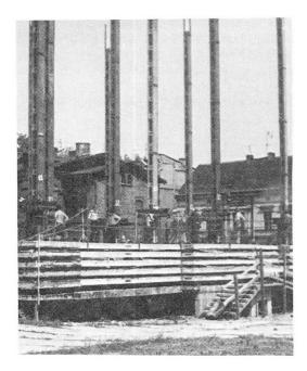
After seating of the last floor slab there follows the disassembly of lifting device and the sliding bars.
