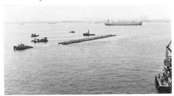
Photo 3 Towing of tunnel element
