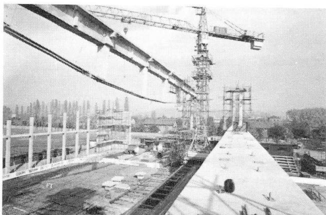
Fig. 1: Lifting of main beams
