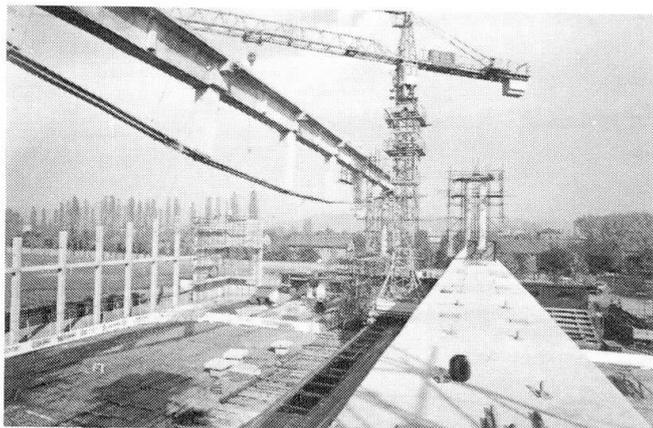
Fig. 1: Lifting of main beams
