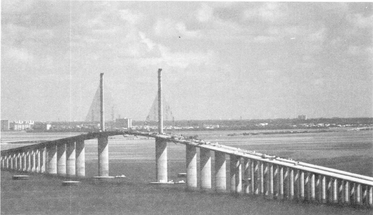
Fig. 11 Placing Last Segment in Main Span
