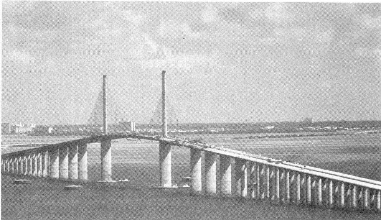
Fig. 11 Placing Last Segment in Main Span
