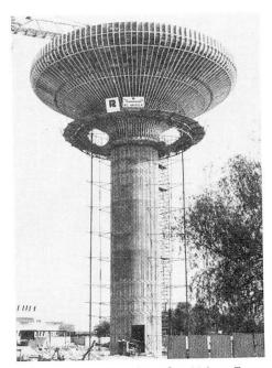
Fig. 1 Formworksystem for Water Tower
