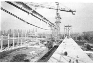
Fig.1: Lifting of main beams
