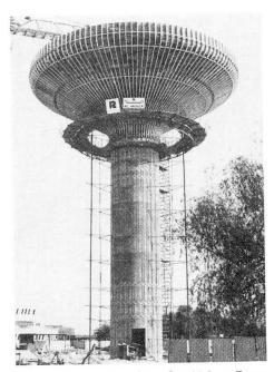
Fig. 1 Formworksystem for Water Tower
