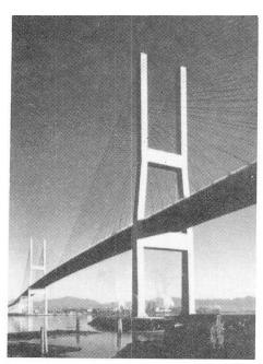
Fig. 17 - Annacis Island Bridge, Vancouver, central span 465 m, composite deck
