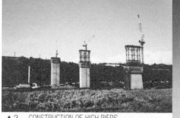
▲ 3. CONSTRUCTION OF HIGH PIERS High piers were constructed by tower cranes and selfclimbing forms. The highest pier is 69.4m. Seismic shaking test was conducted after the completion of piers.
