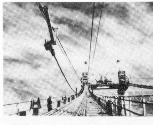
Erection of cable
