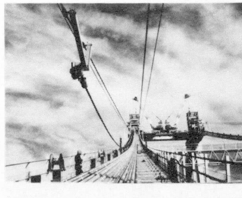
Erection of cable
