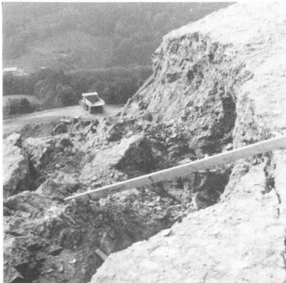
Fig. 5: Loosened Rock Masses Gliding Off. Height of Slope: 50 m
