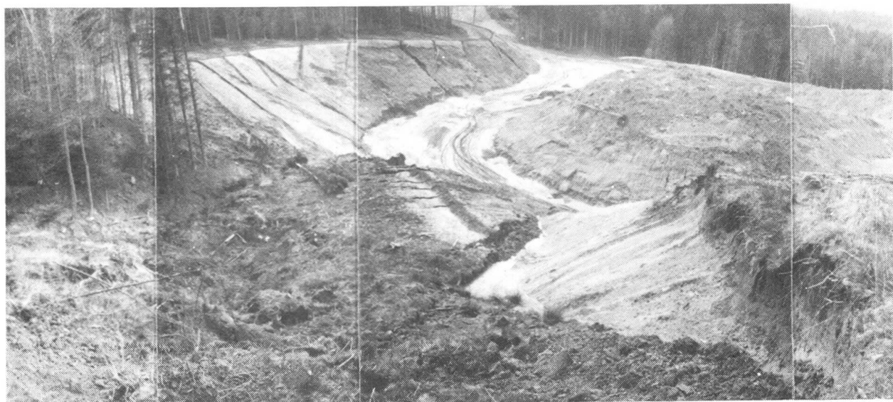
Figure 7 A Rock Mass of 29,000 m 3 Glides Off.
