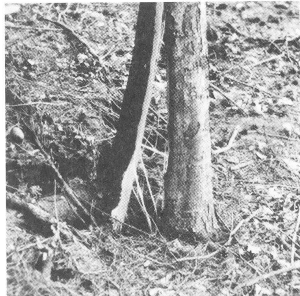
Fig. 6: Crack Above Slope. Width of Crack: 20 cm, Distance to Road: 70 m
