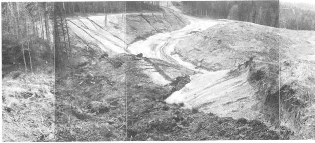
Figure 7 A Rock Mass of 29,000 m<sup>3</sup> Glides Off.
