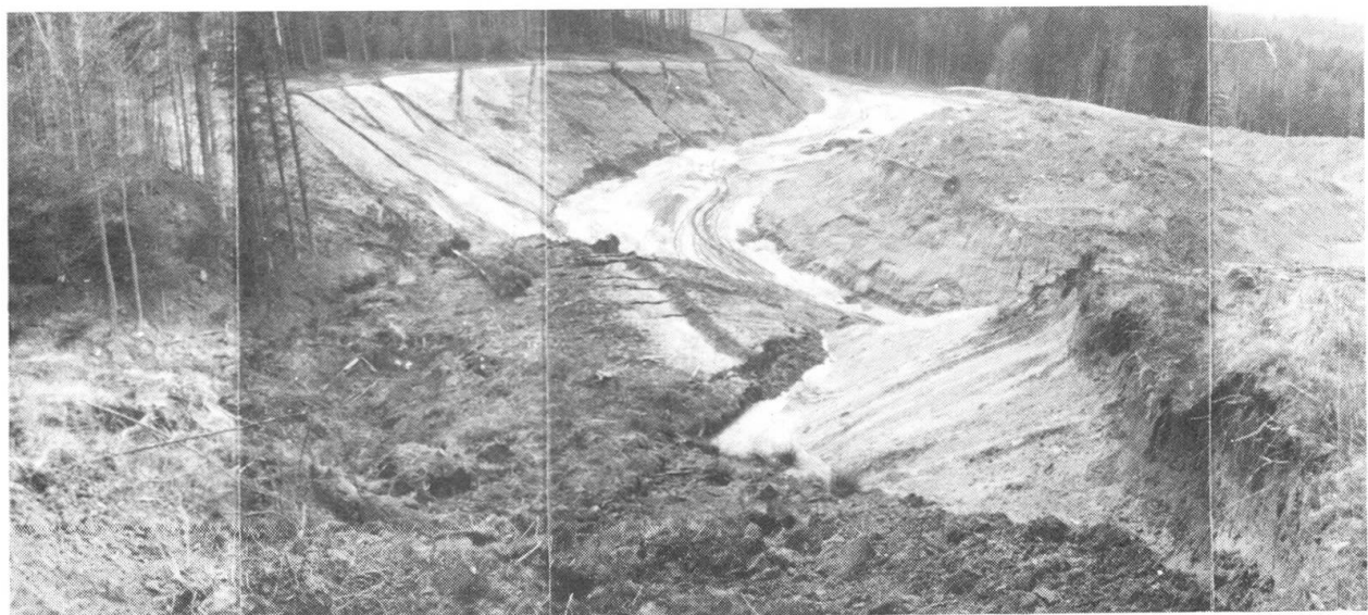
Figure 7 A Rock Mass of 29,000 m 3 Glides Off.
