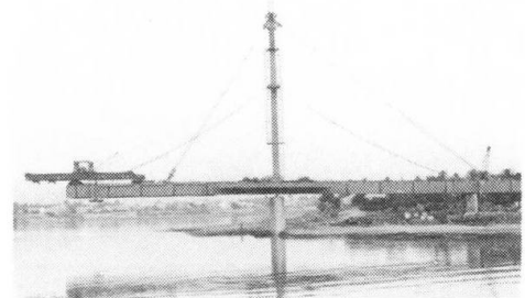
Photo.2 View before the transfer of cable tension
