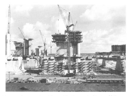
Photo 1 Piers under construction with formwork (Sept. '81)
