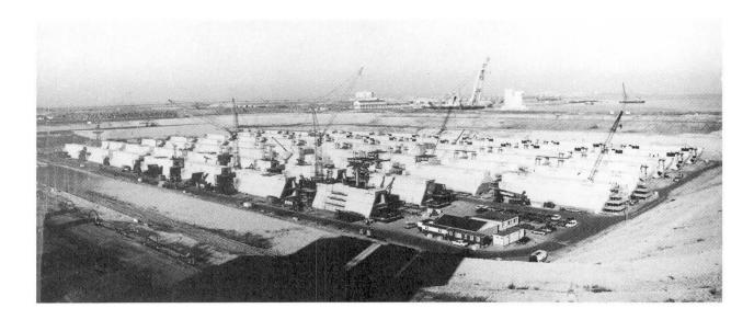
Photo 2 Sill-beams in construction dock (Jan. '85)
