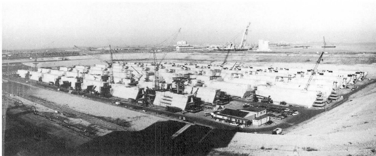
Photo 2 Sill-beams in construction dock (Jan. '85)
