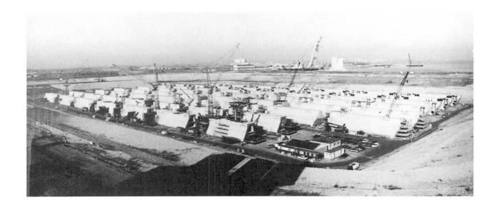
Photo 2 Sill-beams in construction dock (Jan. '85)
