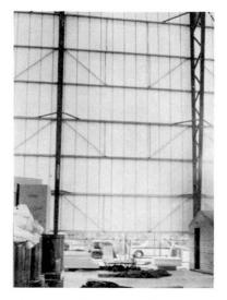
Fig.4. Bracing to sheeting rails
