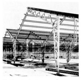
Fig.5. Latticed portal frames - c.1950
