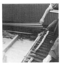
$\underline{\text{Fig. 1}}$  Moisture damaged flat roof with metal sheeting. Moisture penetration from both the inside and the outside. The fibre board hung down, thus blocking the vented air space. The moisture content in the construction increased and caused mould and rot damage. (Example 1.)
