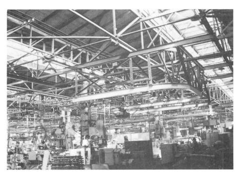
Fig. 3 roof trusses with hanging-crane
