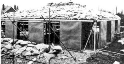
Fig. 2 MACE unit under test
