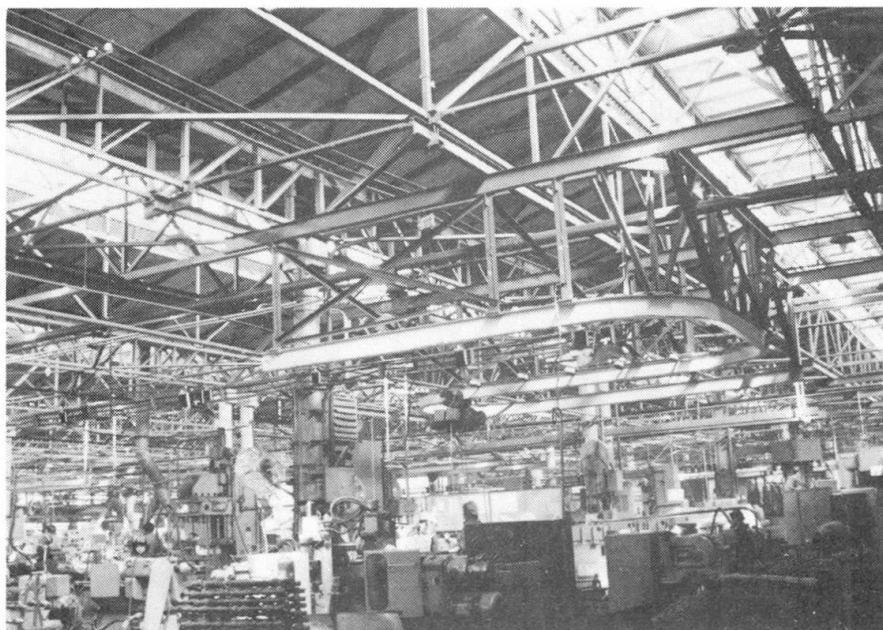
Fig. 3 roof trusses with hanging-crane
