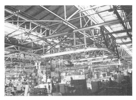
Fig. 3 roof trusses with hanging-crane
