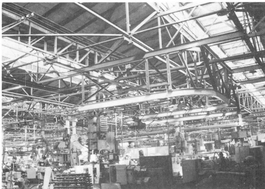
Fig. 3 roof trusses with hanging-crane
