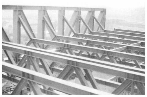
$\underline{\text{Fig. 4}}$  - Transversal reticular girders of the suspension top system.
