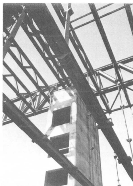
Fig. 5 - Ties and floor beams hanged to the top grid.
