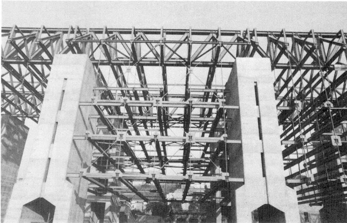
Fig. 6 - Lateral bracings between two towers.
