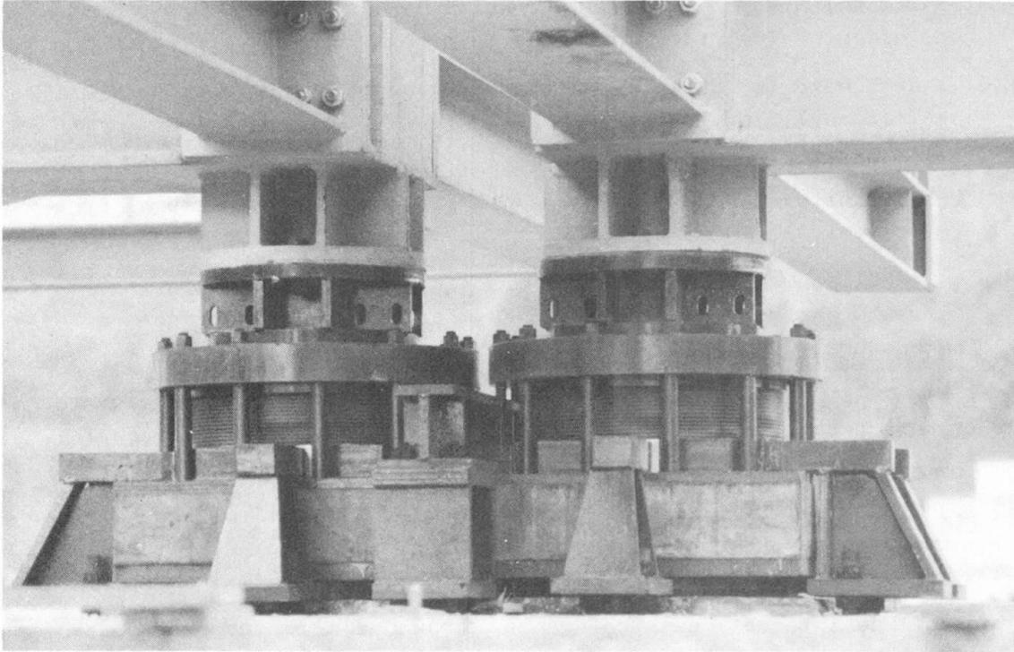
Fig. 7 - Seismic supports of the top grid.
