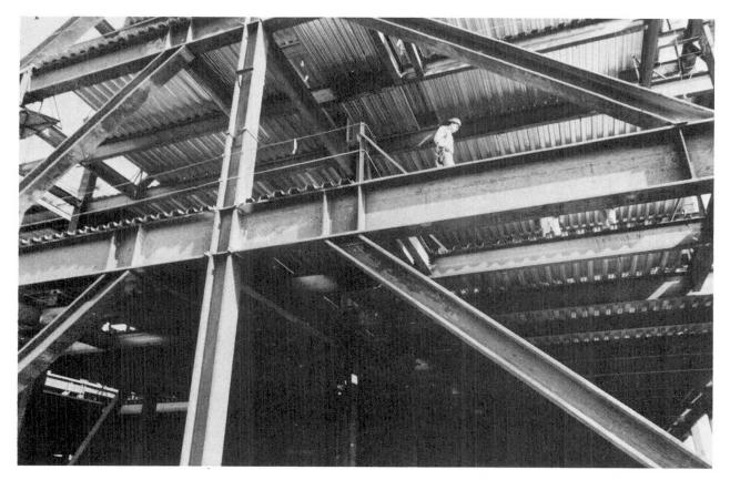
Fig. 3 Eccentric Brace Detail
