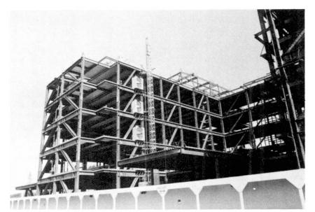
Fig. 2 Eccentrically Braced Frame Hospital
