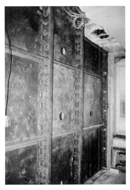
Fig. 4 Steel Plate Shear Wall
