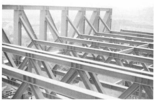
Fig. 4 - Transversal reticular girders of the suspension top system.
