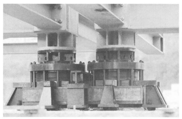
Fig. 7 - Seismic supports of the top grid.
