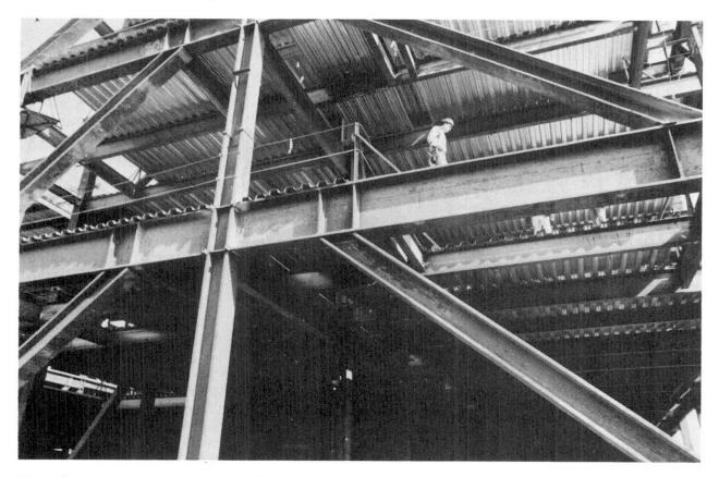
Fig. 3 Eccentric Brace Detail
