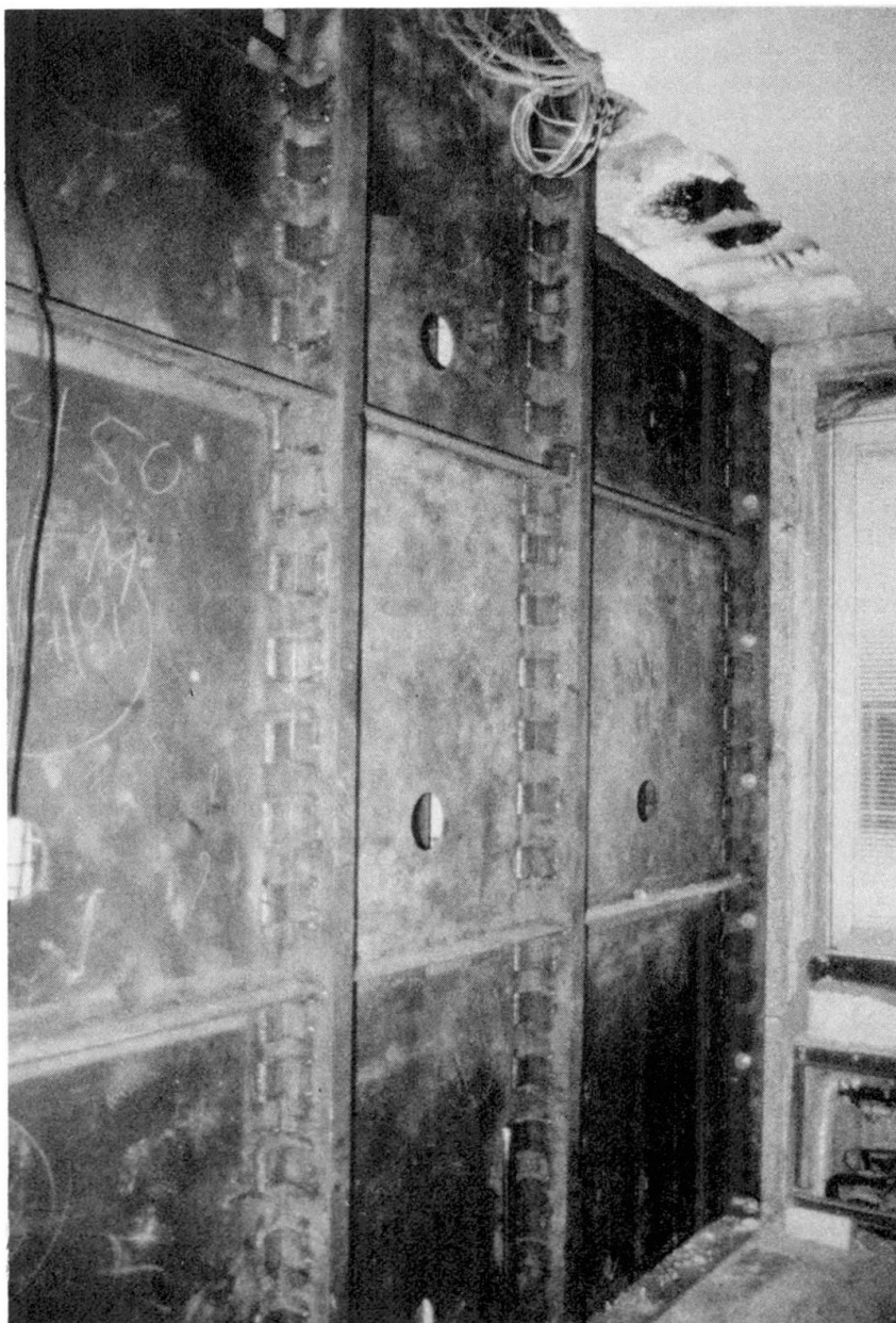
Fig. 4 Steel Plate Shear Wall
