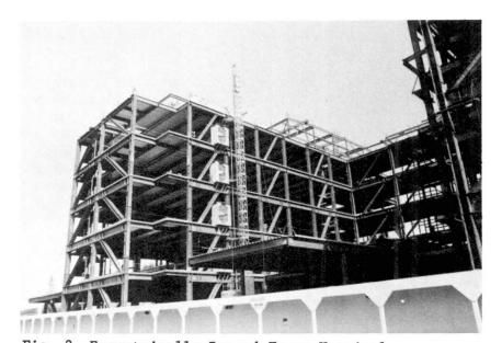
Fig. 2 Eccentrically Braced Frame Hospital
