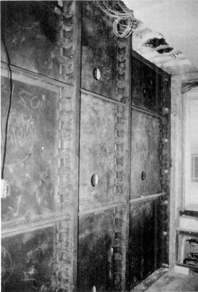
Fig. 4 Steel Plate Shear Wall
