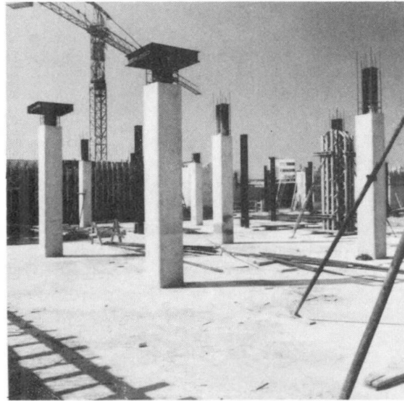
Fig. 6 Composite columns with encased hot rolled H-profiles and steel shear heads: Office building LE FOYER, Luxembourg, 1982
