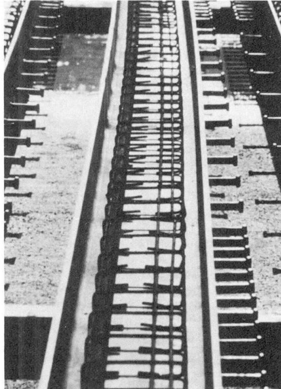
Fig. 2 AF 90 beams before concreting: Office building Magnus Müller, Delmenhorst W-Germany, 1982
