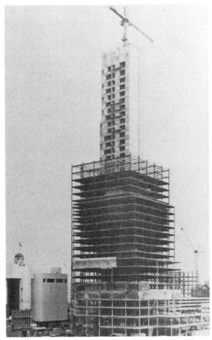
Fig.2 Composite Steel-Concrete Structural System
