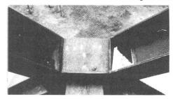
WRONG: Water Trapped in Cross Bracing Connection
