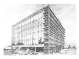
Fig 6 Building "Tour Balexert" at Geneva. All windows and curtain wall in "High Insulation Technology". No heating, only ventilation at 20-22°C.
