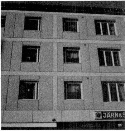
Fig. 6 Steel sheet units are similar to rendering
