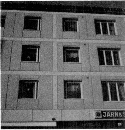
Fig. 6 Steel sheet units are similar to rendering
