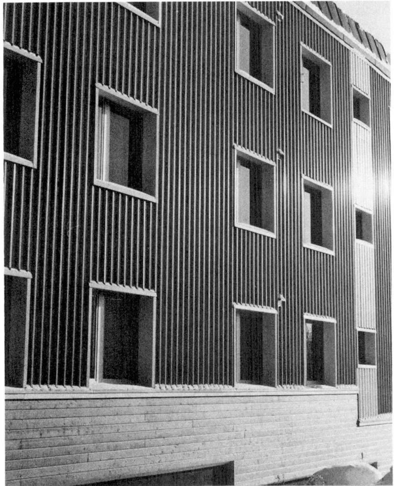
Fig. 7 A base clad with woodpanels is more resistant against damages than steel sheet
