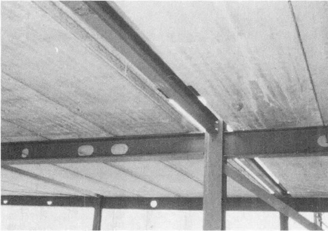
Pre-cast concrete floor design giving uninterrupted service zone
